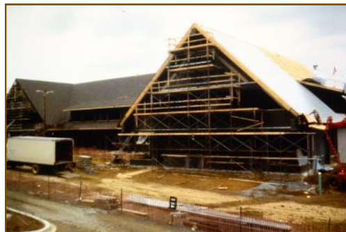
Arsht Hall under construction Scanned by Lee Kaser from a slide by Glen Barbaras
